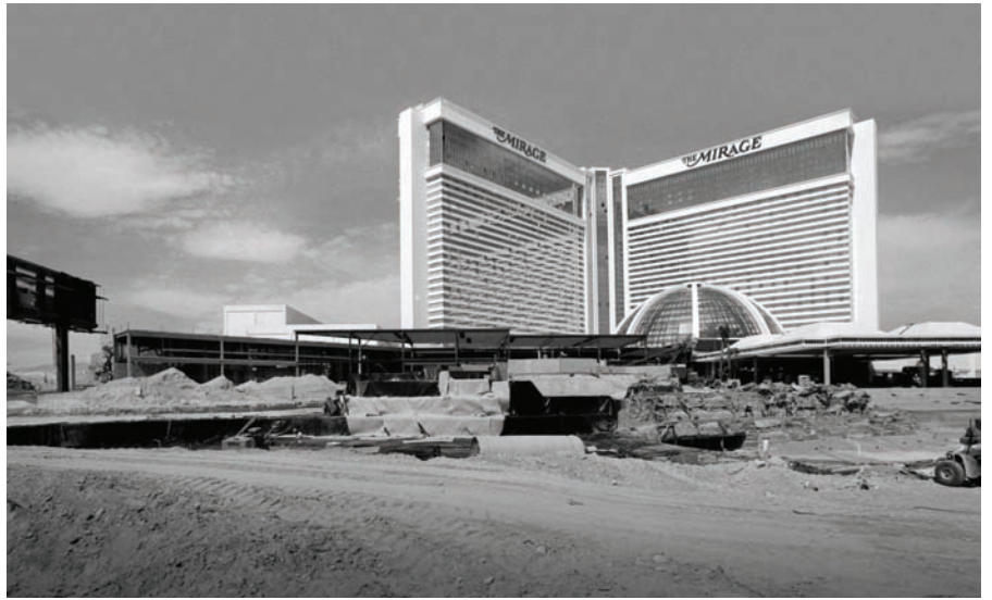
The Mirage under construction
